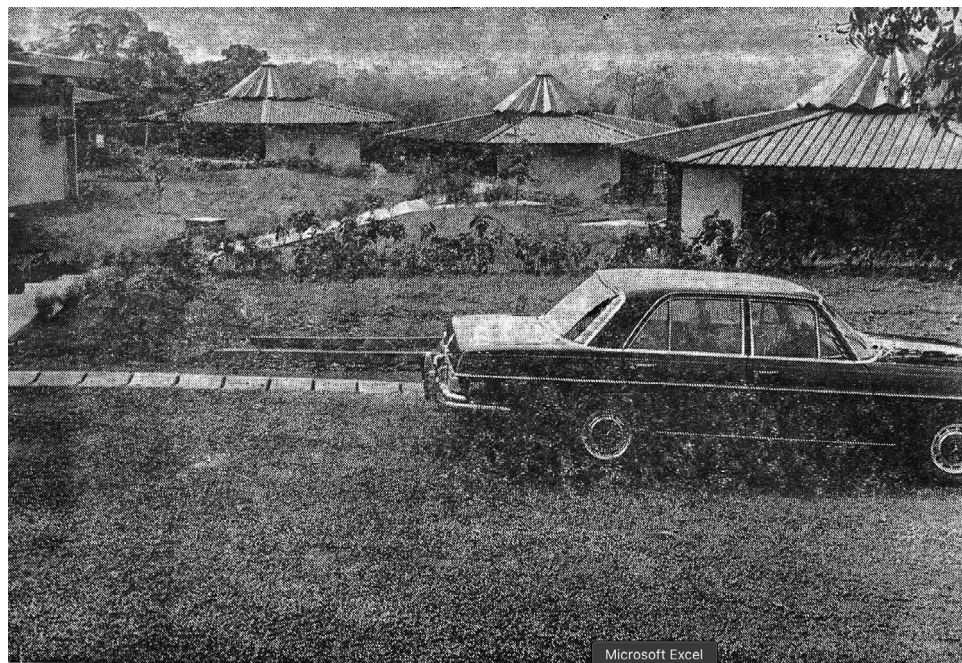
Figure 1: IRIC buildings on the campus of the University of Yaoundé 6 (source: IRIC Brochure, Graduate Institute Archive, Geneva, HEI 2431; reproduced by permission of the International Relations Institute of Cameroon)
