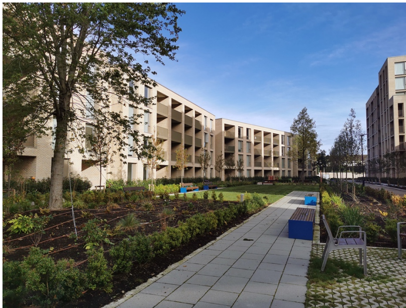
Figure 4.11: Hamilton Gardens apartments façade and green area. Source: Mandy O'Neill, October 2023.
