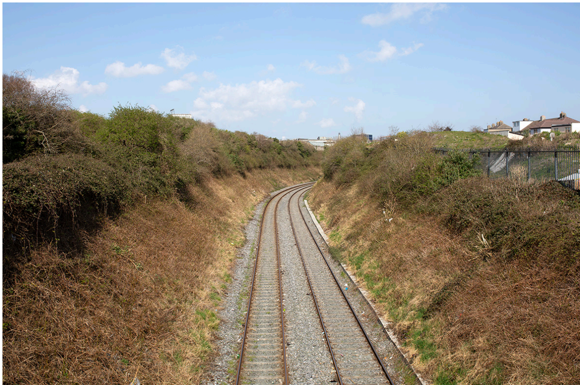
Figure 6.26: Photograph of railway at Fassaugh Avenue Bridge. Source: Mandy O'Neill, 2021.
