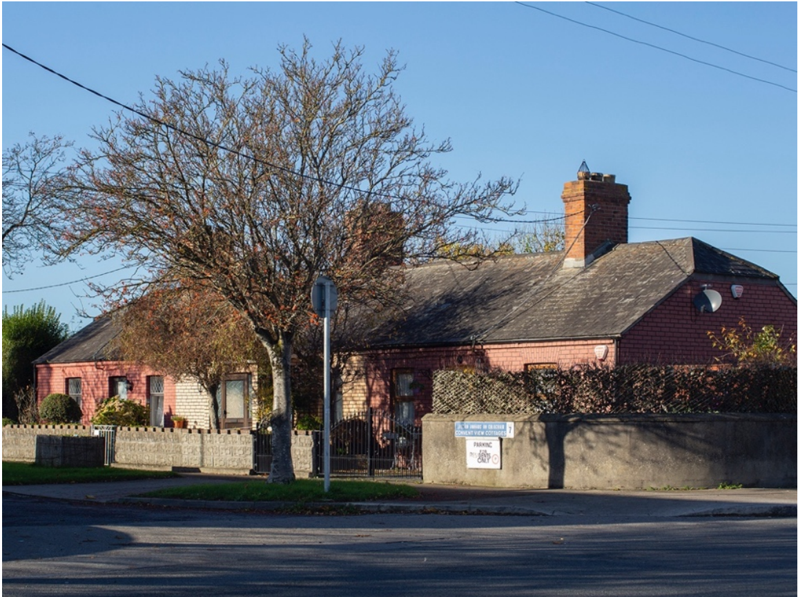
Figure 1.8: Example of early 20 th century housing at Convent View cottages, Ratoath Road, Cabra. Source: Mandy O'Neill, 2020.
