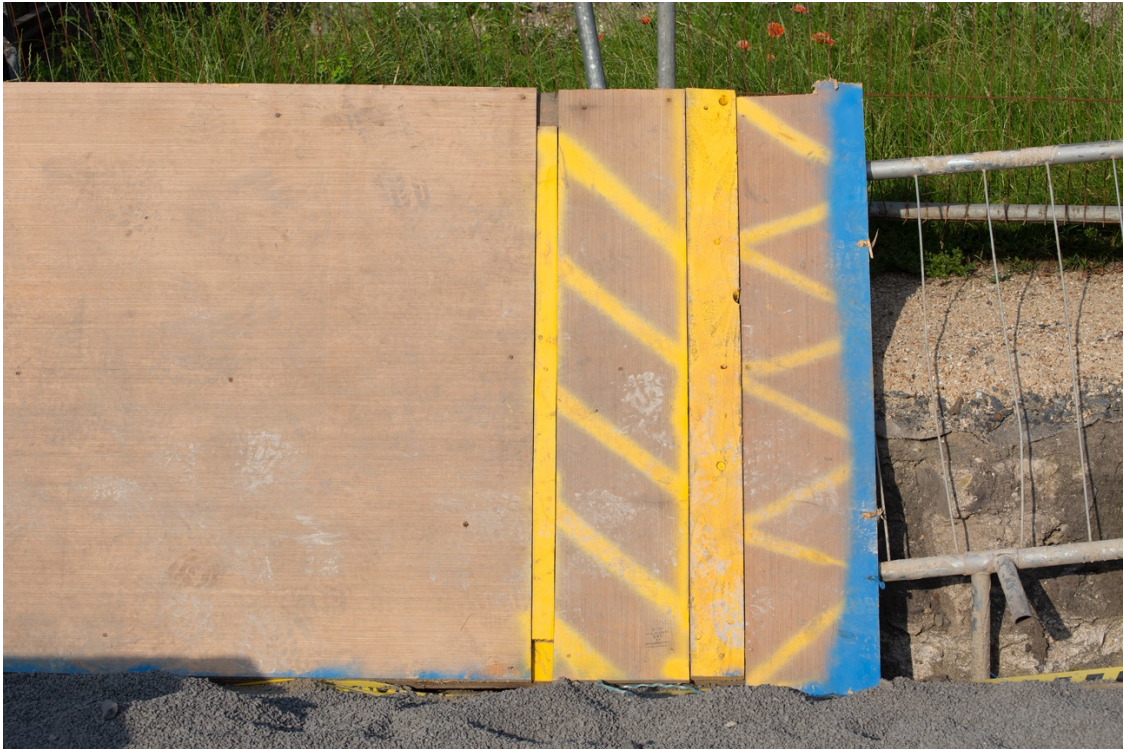
Figure 6.13: Photograph of Hamilton Gardens building site. Source: Mandy O'Neill, 2021.
